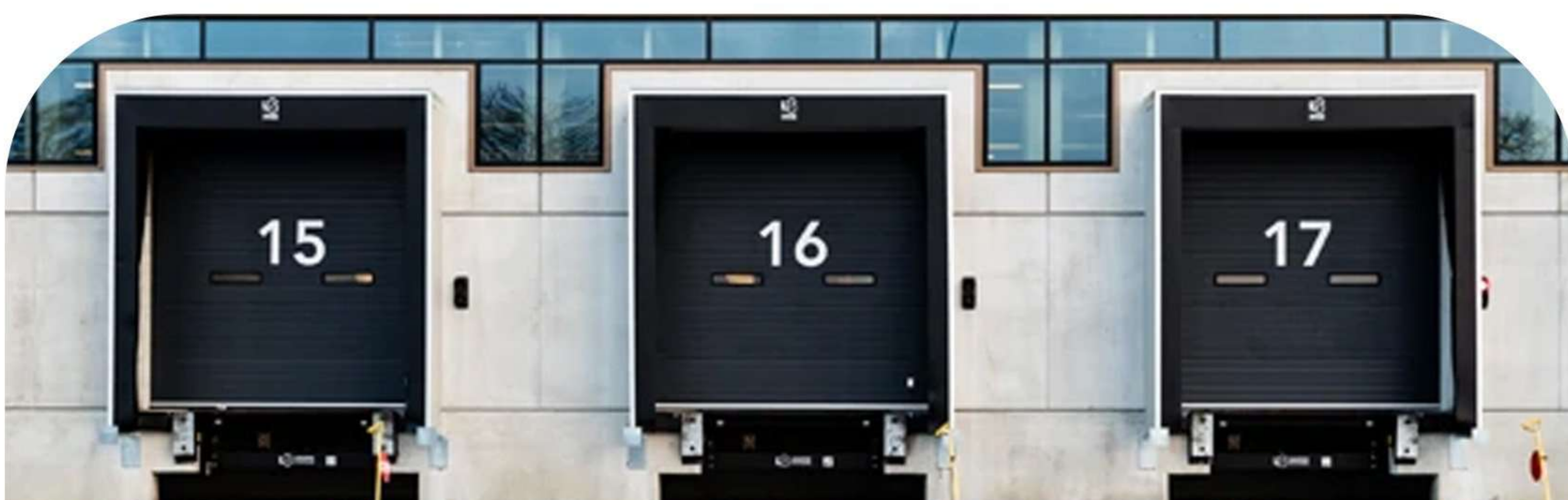
DOCKING BAY & WAREHOUSE SOLUTION
